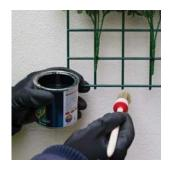
STEP 4 Protect cut point with metal paint.
